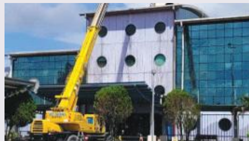
VTMS radar tower installation in progress at Senari Terminal.
