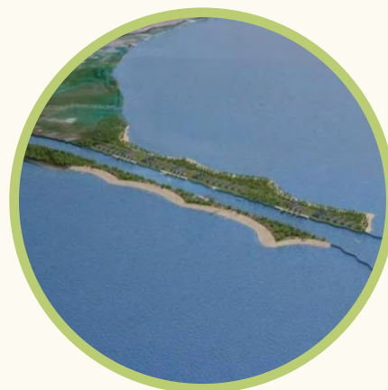
Initial land formation together with access channel dredging works
