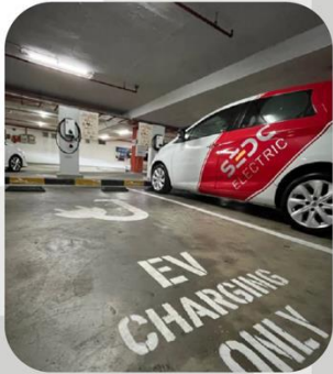
Location: UTC Sarawak Installed Equipment: 2 x 22kW AC Charger
